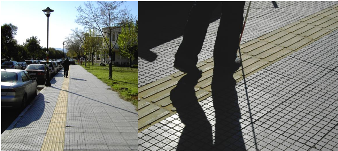
Figure 3: TSI (Tactile Surface Indicator) along pedestrian route and sidewalk Implementation of TSIs at the Aristotle University of Thessaloniki
